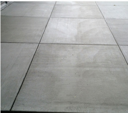
Reinforced Concrete Slab
