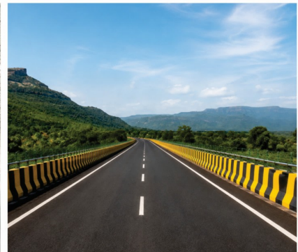
Highway Crash Barrier
